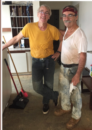
John Alberts and Mike Lallave removing flood-damaged carpet from the 2UC office.
